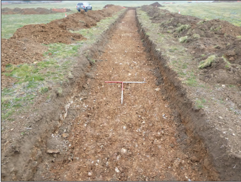
View of trench 34, looking east (1m scales)
